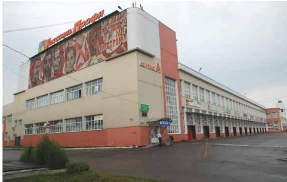
Fig. 1. The Spinning building of the factory "Krasnaya Talka" [9]
