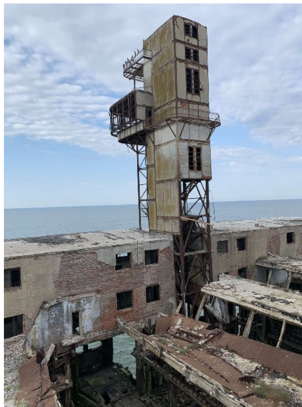
Fig. 3. Observation tower of Dagdiesel Factory no. 8 (2022, photo by the author)
