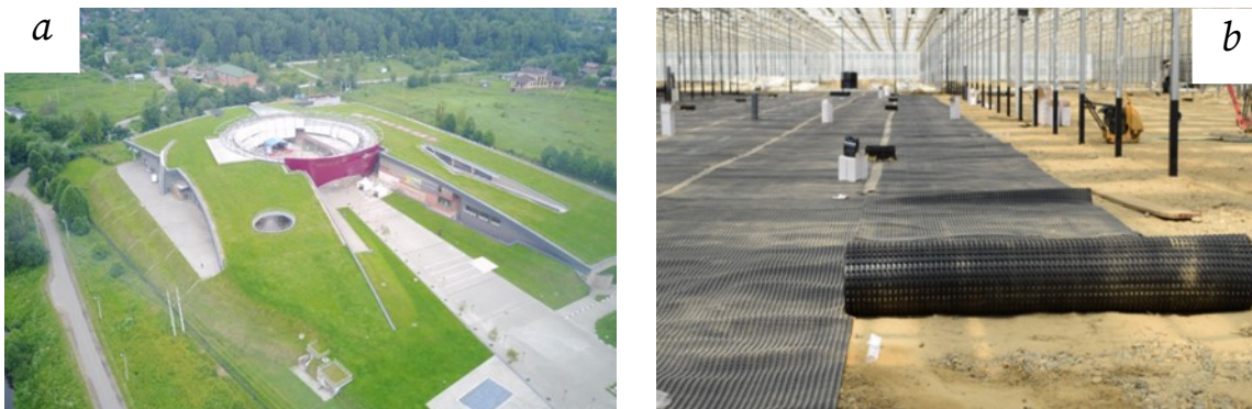
Fig. 6. Application of profiled membranes at real construction objects: a – the green roof of the museum complex; b – installation of floors on grade for a large agricultural complex
